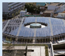
Photovoltaic power generation panels
