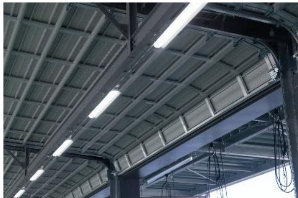
LED lighting (installed in all fixtures)
